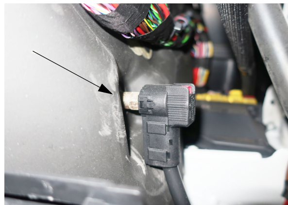
Chassis Battery Connector (Located to the right of the accelerator pedal inside access panel)
