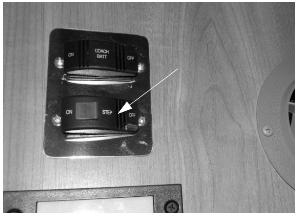
Entry Step Switch (Located near entrance door)
