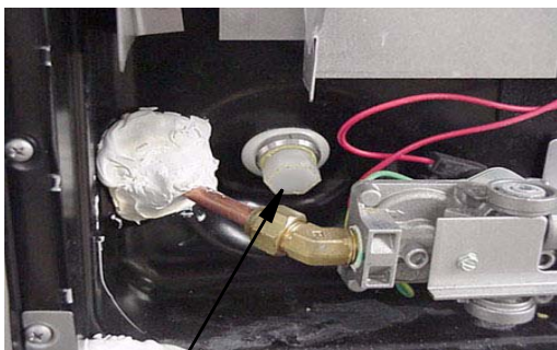
Water Heater Drain Plug Remove with socket.
