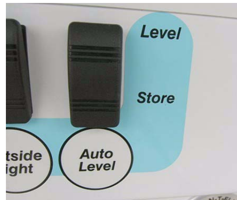
Auto Level Switch in Service Center compartment
