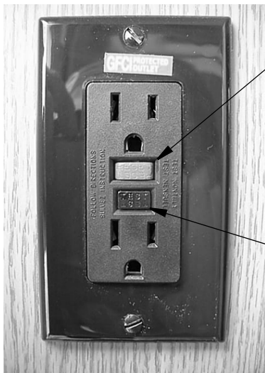
GFCI Outlet (Ground Fault Protector)
