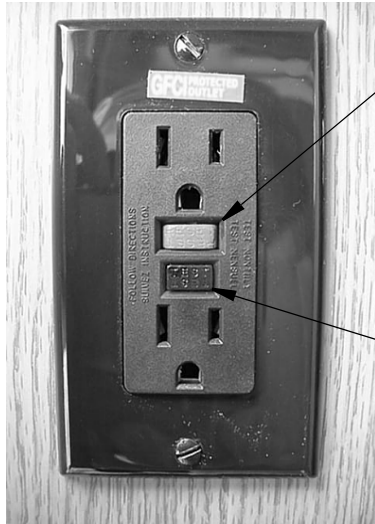
GFCI Outlet (Ground Fault Protector)
