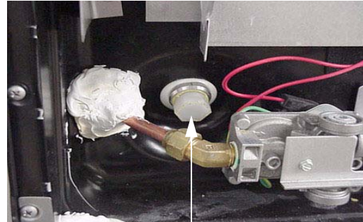
Water Heater Drain Plug (Remove with socket)
