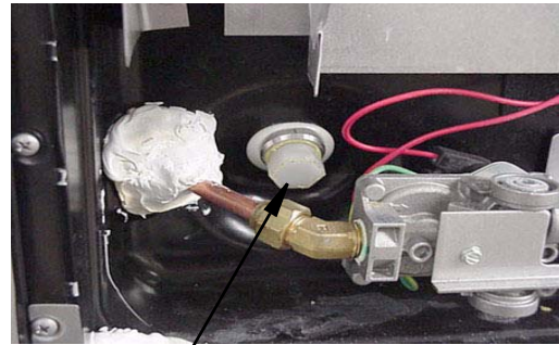
Water Heater Drain Plug Remove with socket
