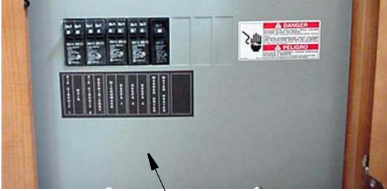
110-Volt Circuit Breakers Shown for Models 33L, 34A, 35N
