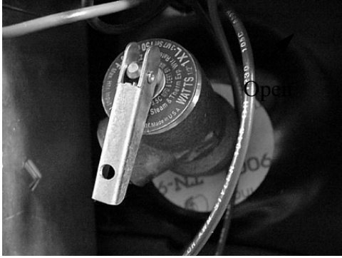
Lift handle straight out to open P-T valve
