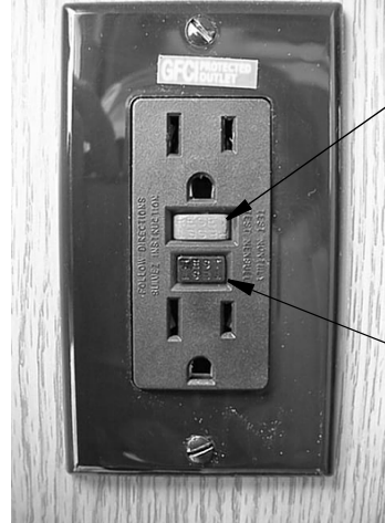
GFCI Outlet (Ground Fault Protector)
