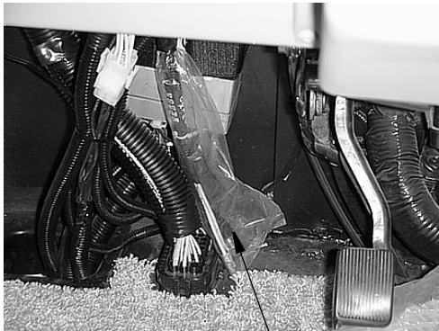
CB Power Wires (in plastic sheath)
