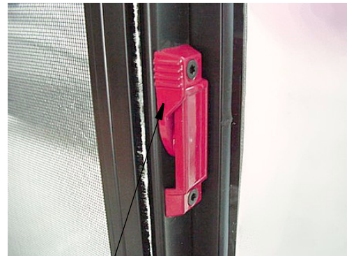
Pull latch outward to slide window open
