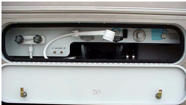
Water Service Center
