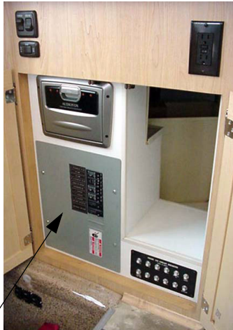
110-Volt House Circuit Breakers
