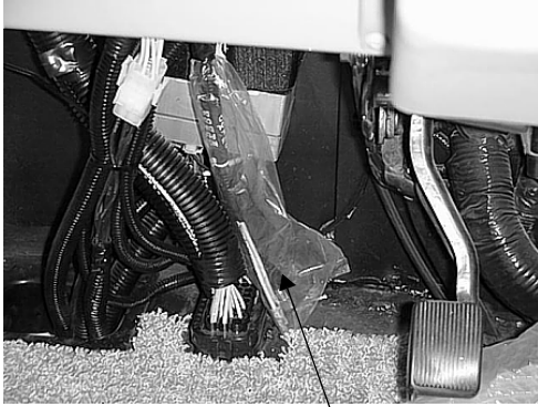
CB Power Wires (in plastic sheath)
