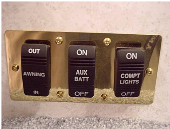
Aux. Batt. Switch (near entrance door)
