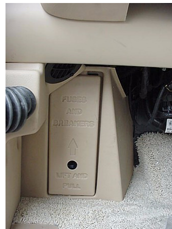
Automotive Fuse/Breaker Panel (In Front of Driver’s Seat)
