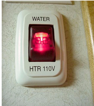
Electric Water Heater Switch (Typical)
