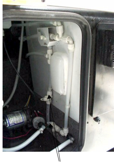
Water Line Drain Valves (in water pump compartment)
