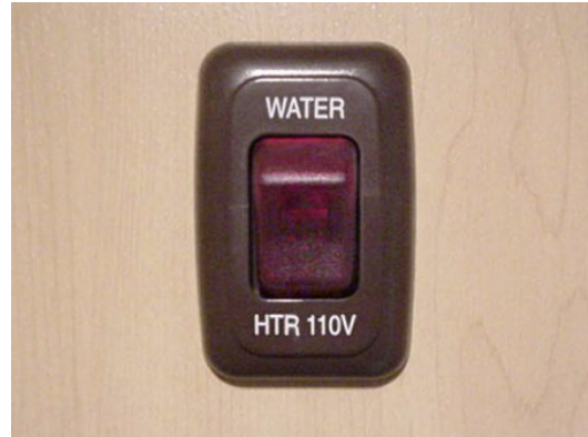
Electric Water Heater Switch (Typical)
