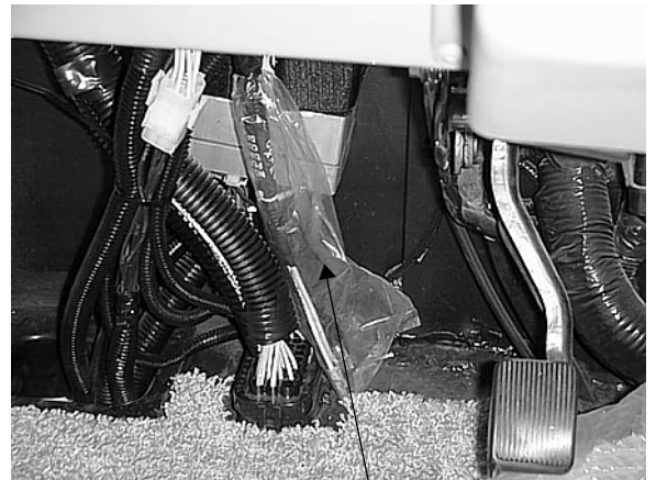
CB Wires (in plastic sheath)
