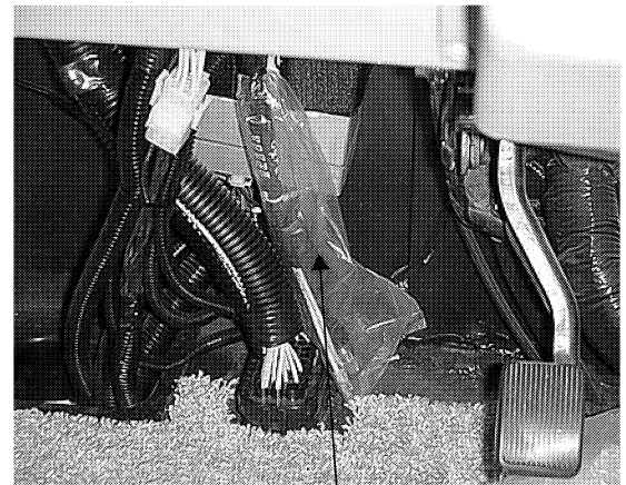
CB Wires (in plastic sheath)
