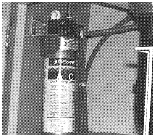
Water Filter Assembly - Below Galley Sink
