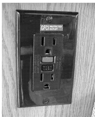
GFCI Outlet (Ground Fault Protector)
