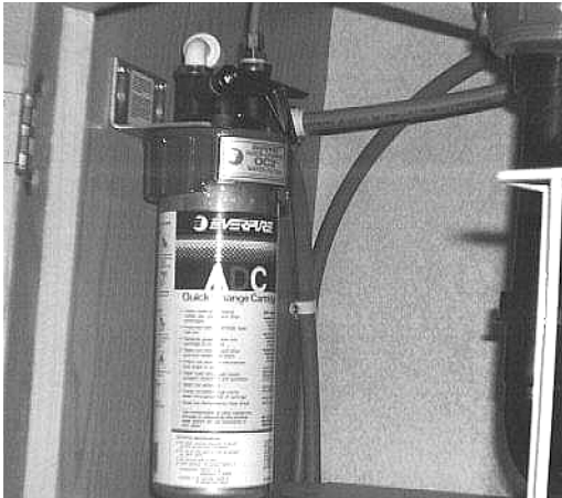
Water Filter Assembly - Below Galley Sink
