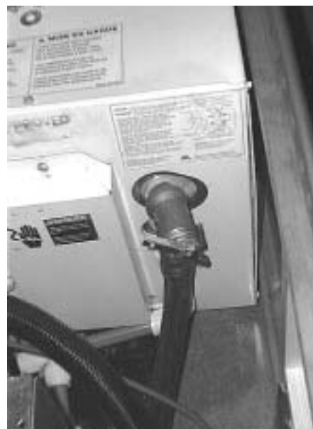
Pressure-Temperature Relief (P-T) Valve
