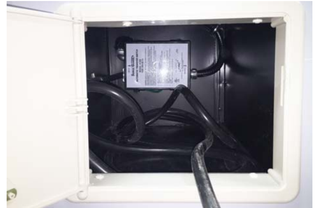
Automatic Power Transfer Box (Located inside utility compartment) -Typical installation shown
