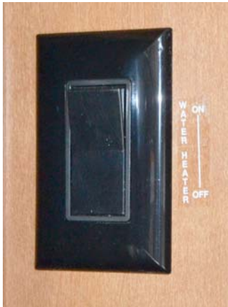
Electric Water Heater Switch (Typically located near Systems Monitor Panel)
