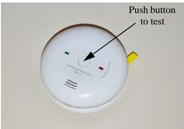
Carbon Monoxide Alarm
