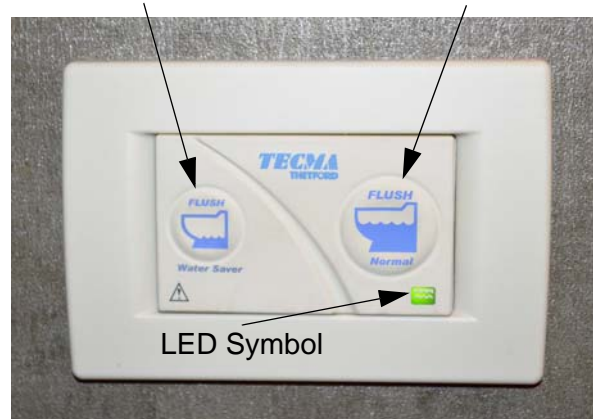
Wall Switch/Controller (Located on wall near toilet)
