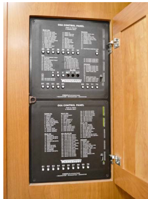
House Circuit Breakers -Typical View
