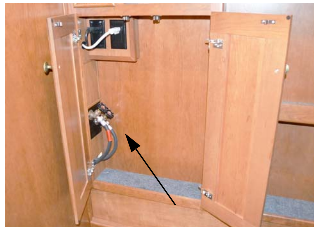
Water Supply Faucets (Located inside bathroom wardrobe cabinet) *Model 45RL
