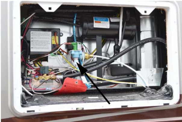
Ice Maker Water Supply Connection -Typical View
