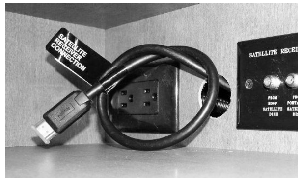
HDMI Cable (Located in a front overhead cabinet) -Typical View
