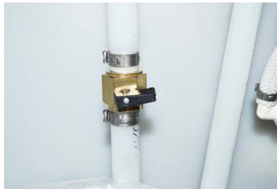
Water Tank Drain Valve -Typical installation shown
