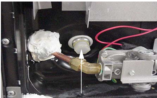
Water Heater Drain Plug (Remove with socket)
