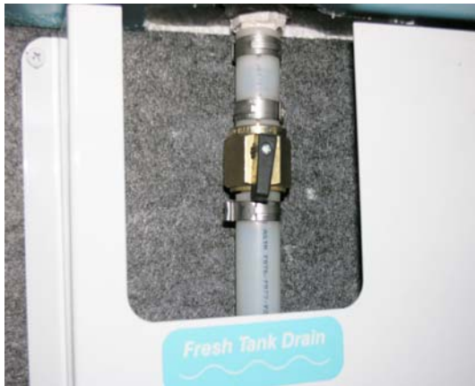
Water Tank Drain Valve -Typical Installation
