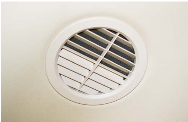
Return Air Vent (Grasp louvers and pull straight down to remove air vent) -Typical View
