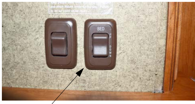
Power Lift/Lower Control Switch (Located near bedroom nightstand) -Typical View
