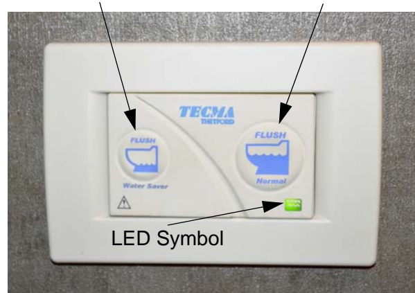
Wall Switch/Controller (Located on wall near toilet)
