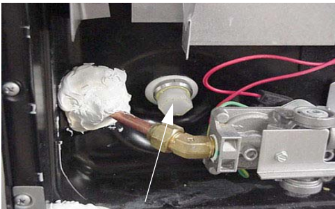
Water Heater Drain Plug (Remove with socket)
