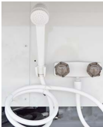
Exterior Shower/Wash Station -Typical View
