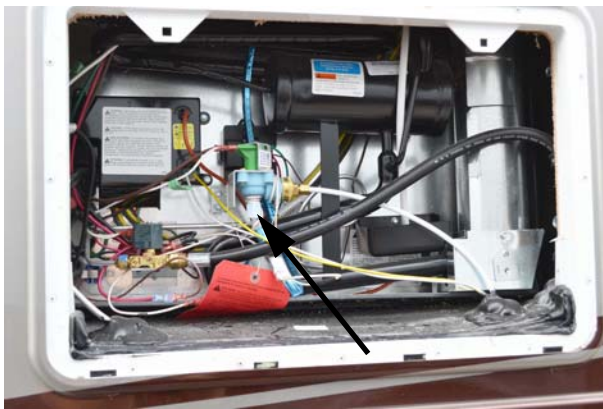
Ice Maker Water Supply Connection (Located in refrigerator service access compartment on outside of coach) -Typical View
