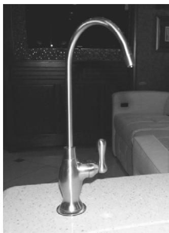
Filtered Water Faucet -Typical View
