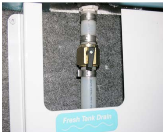
Water Tank Drain Valve -Typical Installation
