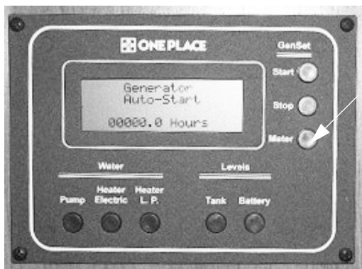
Generator Hourmeter Button -Typical View
