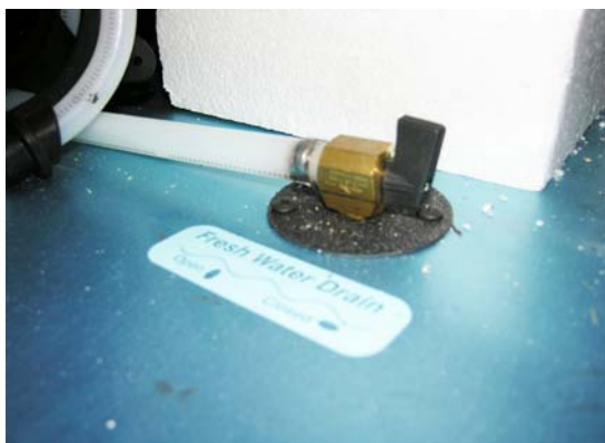
Water Tank Drain Valve -Typical Installation
