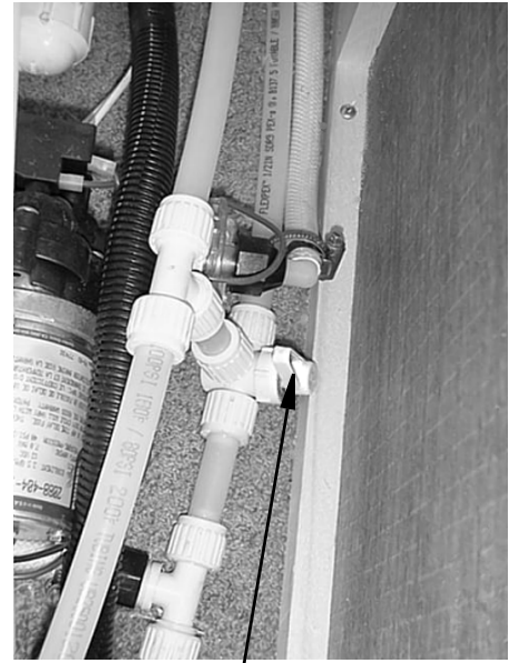
Waterline Drain Valve (Typical)
