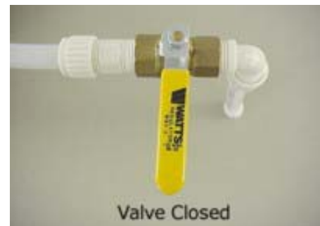
Water Tank Drain Valve (Typical)
