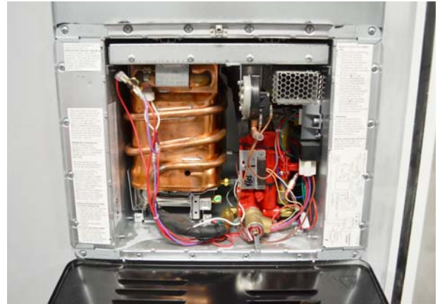
Water Heater Exterior Service Access -Typical View
