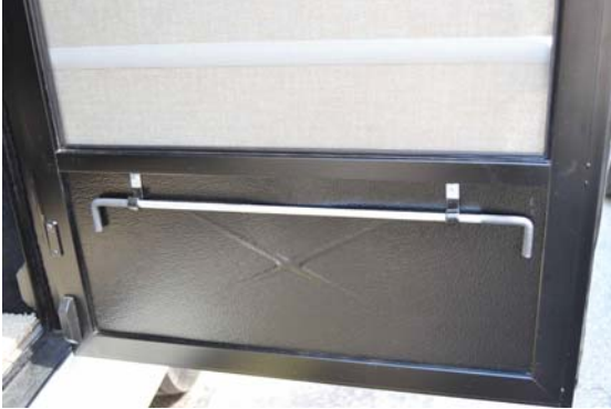
Prop Rod Storage Location (Located on inside of screen door) -Typical View
