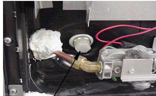
Water Heater Drain Plug (Remove with socket)
