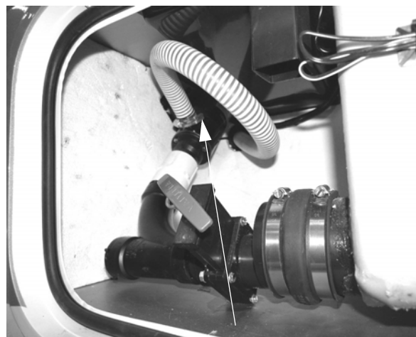
Waste Pump (Located in driver side compartment behind rear wheel)
