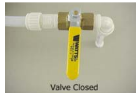
Water Tank Drain Valve -Typical Installation
