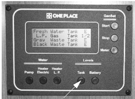
Tank Levels Switch
