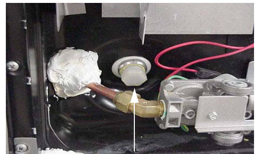
Water Heater Drain Plug (Remove with socket)
