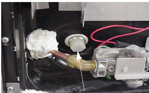
Water Heater Drain Plug (Remove with socket)
