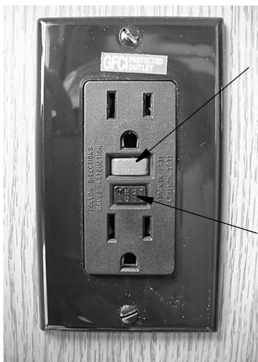
GFCI Outlet (Ground Fault Protector)
