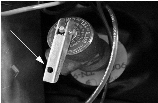
Pressure Temperature Relief Valve (Lift handle only when water heater is cold)
