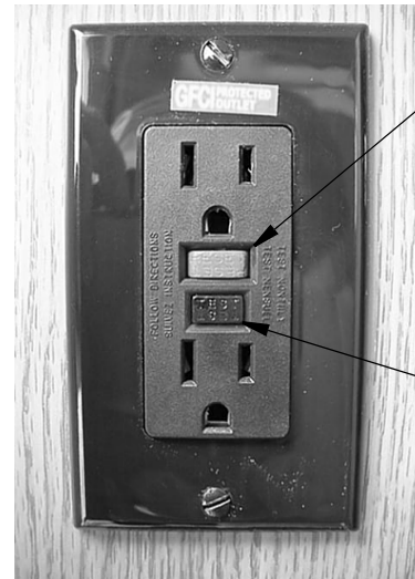
GFCI Outlet (Ground Fault Protector)
