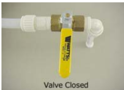
Water Tank Drain Valve (Typical) Under Rear Bed or Couch
