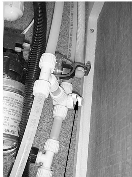
Waterline Drain Valve (Typical)
