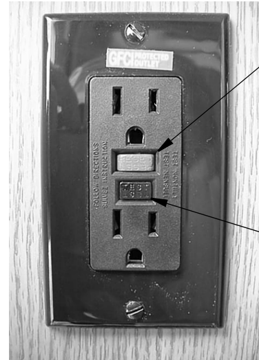
GFCI Outlet (Ground Fault Protector)
