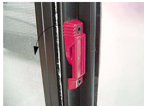
Pull latch outward to slide window open
