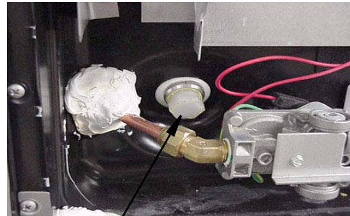
Water Heater Drain Plug Remove with socket.
