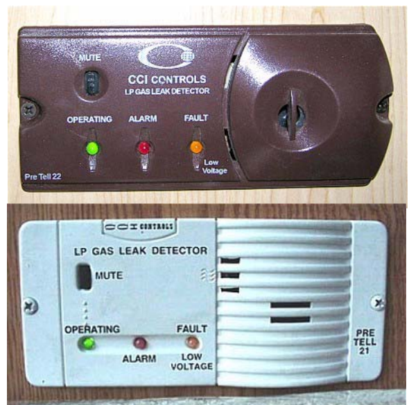
Propane Gas Leak Detectors (typical)
