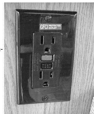
GFCI Outlet (Ground Fault Protector)
