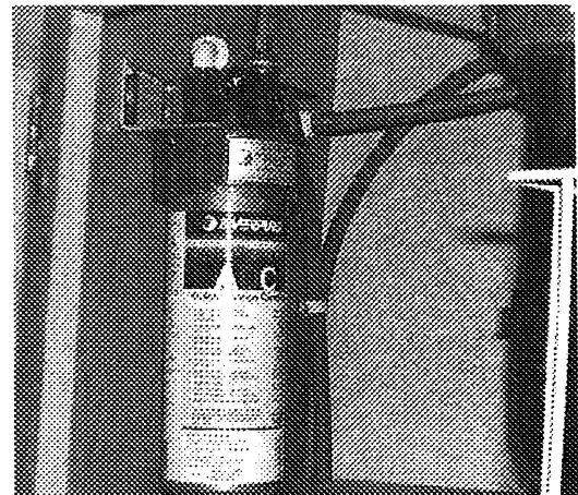
Water Filter Assembly - Below Galley Sink
